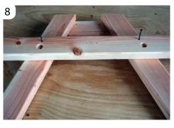
Place a flat washer, split-lock washer, and nut on each carriage bolt and tighten securely, but be sure not to over-tighten. Repeat for the other leg brace/leg support assembly.
