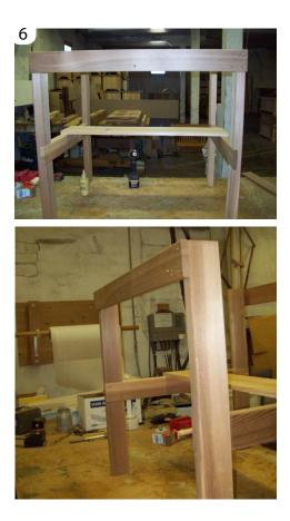
Turn the leg section on its side with the top facing you. Find the  $1 \frac{1}{4}$ " W x 30  $\frac{1}{4}$ " L piece and install it in between the upper leg section with the rounded side facing up. It should fit tight. Attach using  $1 \frac{1}{2}$ " screws. Repeat on other side.
