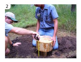
Make sure each log step is level and plumb in the footings, as well as the proper distance apart from each other. You may need to fill the holes with additional material as needed to fit post.
