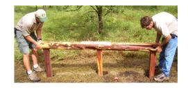
Make sure that the highest designated play surface is the proper height. Also check to see that the beam is level and plumb in footings. You may need to fill the holes with additional material as needed to fit post.
